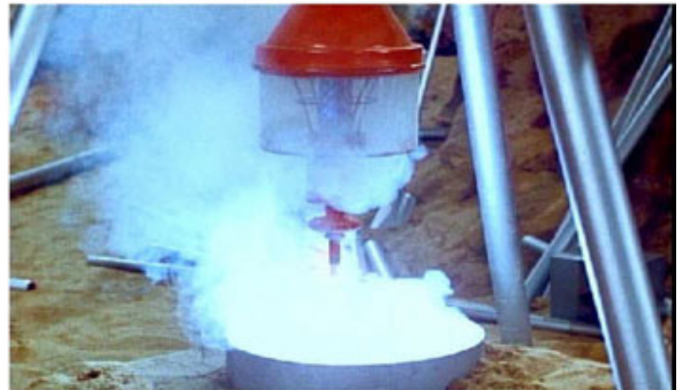
Drilling Rig in Operation
